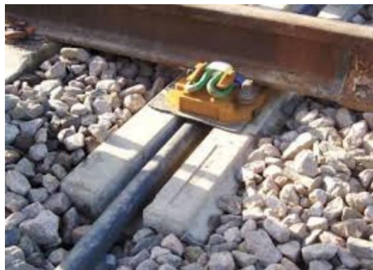
Plate 1. Concrete hollow sleepers
